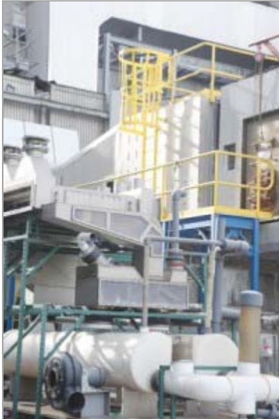
The Neustream, pictured above, is 90 percent smaller than conventional scrubbers. The smaller size allows Colorado Springs Utilities to continue using the aging Drake power plant.
